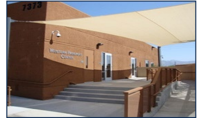
U.S. Dept of State/Bureau of Consular Affairs/Western Passport Center ±76,268 SF Tuscon, AZ
