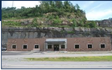
Mine Safety & Health Administration ±12,994 SF Logan, WV
