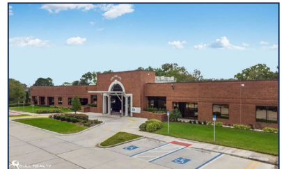
Sabal Park Clinic ±44,099 SF Tampa, FL
